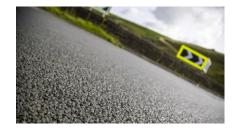
✓ The Border Road Organization (BRO) has planned to build steel slag road in Arunachal Pradesh on a pilot project basis. The Steel Slag Road, which can survive heavy rain and difficult weather conditions, is the first of its kind project of the BRO. This Road project will help to connect the strategic locations in the Northeast India.
